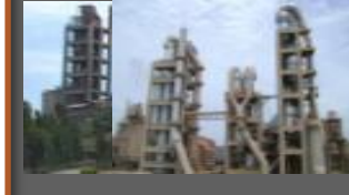
Line - III commissioned
